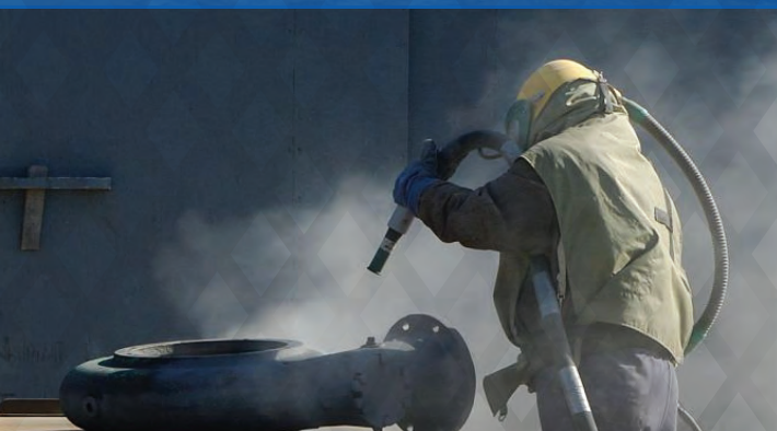
Sand Blasting & Painting
